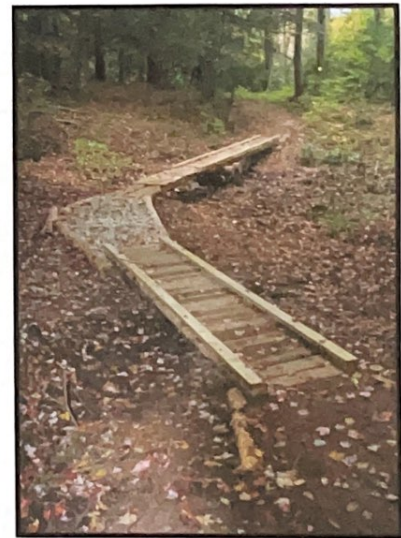
Puncheon, or wooden walkway, constructed on Allegheny Trail in Canaan Valley State Park
